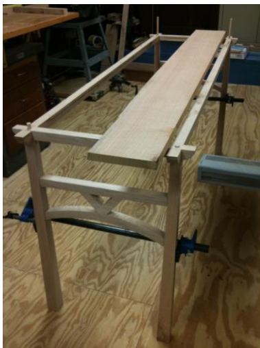
Figure 3. Frame and legs assembled with ornamental piece.
